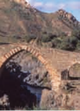
Saracen bridge, Adrano (CT)
